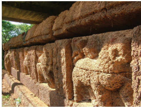
Fig.2 The laterite base of Hsinday Myindat, decorated with the series of lions and elephants in square panels
